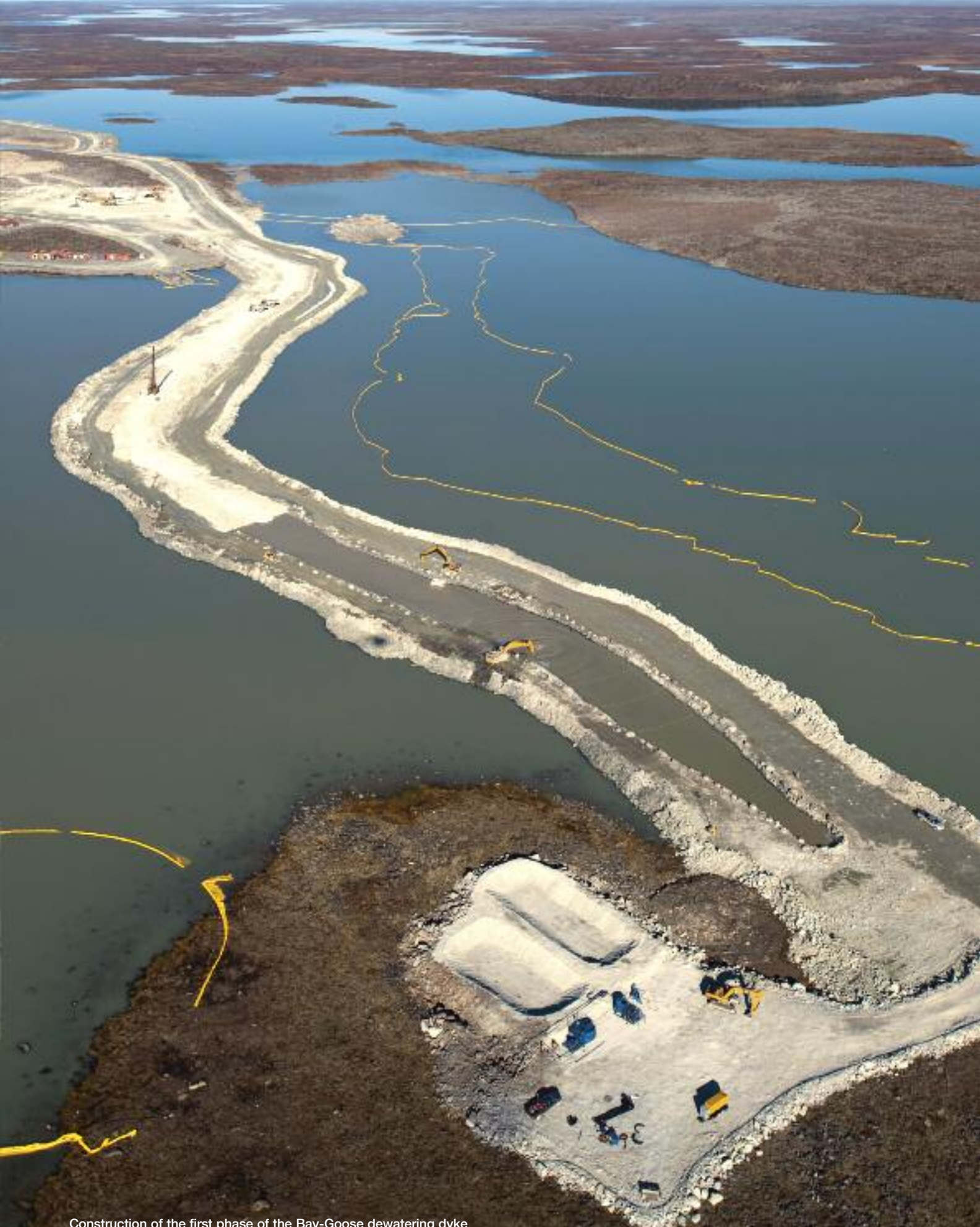
Construction of the first phase of the Bay-Goose dewatering dyke at the Meadowbank mine – Summer of 2009
